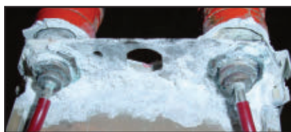
▲ Fig. 2 Effect of galvanic corrosion.
